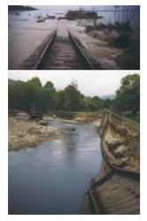
Figure 3 - Railway destroyed by flood
