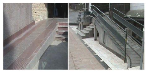
Picture 4: An entrance to a general hospital, the slope of ramp is not standard and is unprotected border. Picture 5: Ramp of inappropriate slope for access into a clinic.
