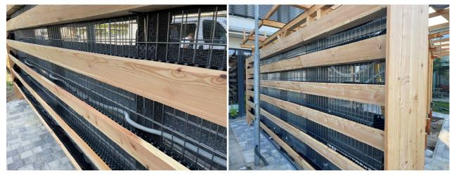
Fig. 9 and 10: Ground construction/substructure of the EVAPO+ transpiring green wall within the outdoor classroom at the Middle School in Strasshof
